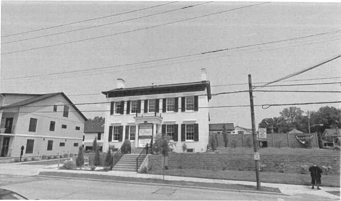
Image 1: Benjamin Stewart House located at 5540 Madison Rd. Image provided by applicant.
