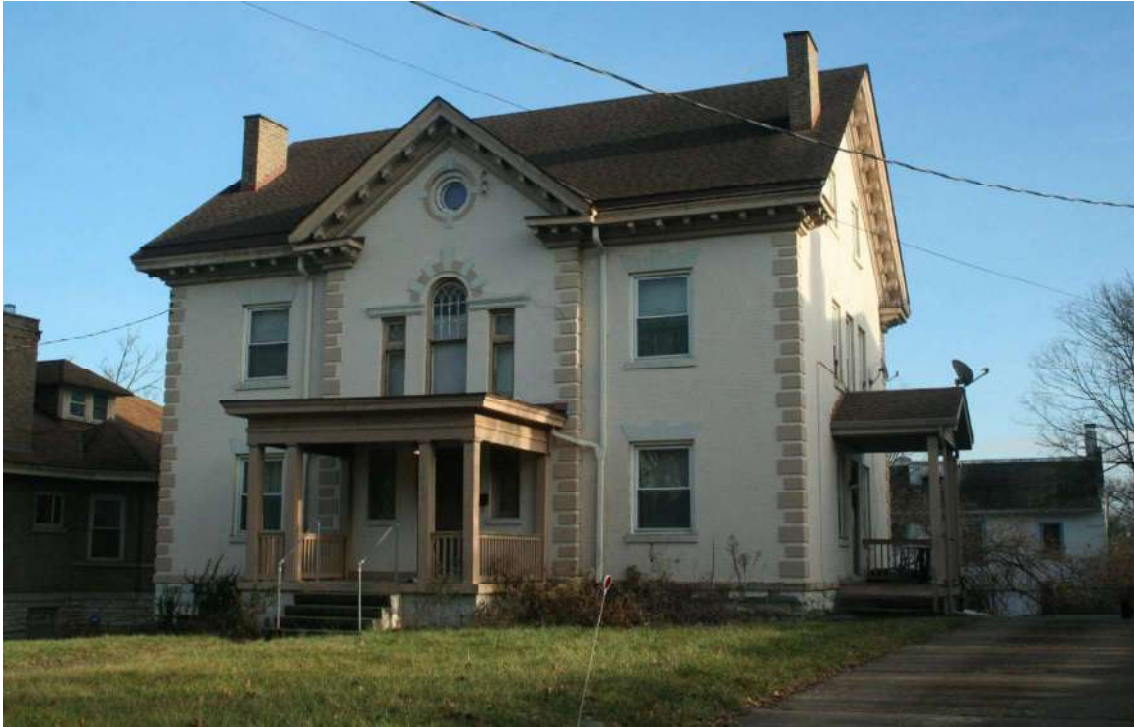
Photo 26. 3818 Dakota Avenue (1920), Georgian Revival.
