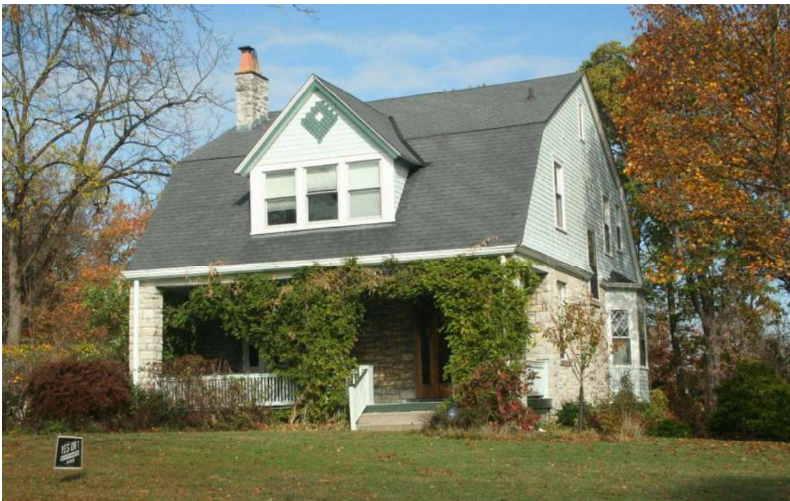
Photo 25. 978 Avondale Avenue (1913), Dutch Colonial.
