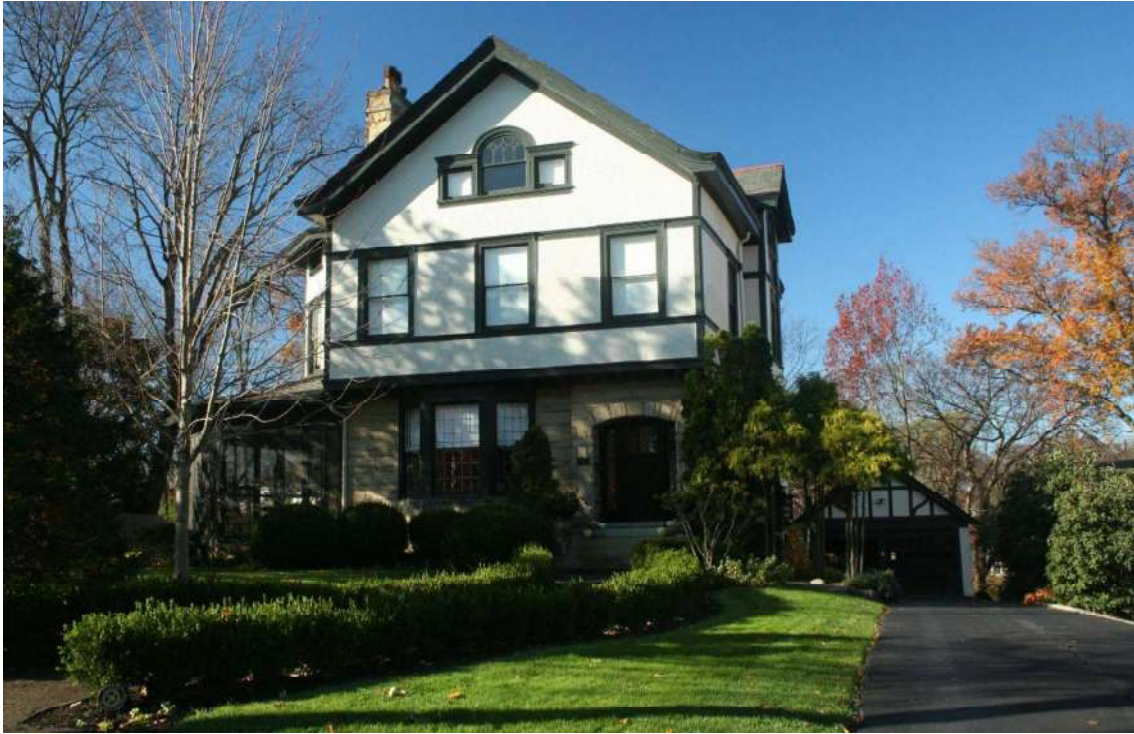
Photo 8. 3971 Beechwood Avenue (1898), Charles H. Ferber, Eclectic.
