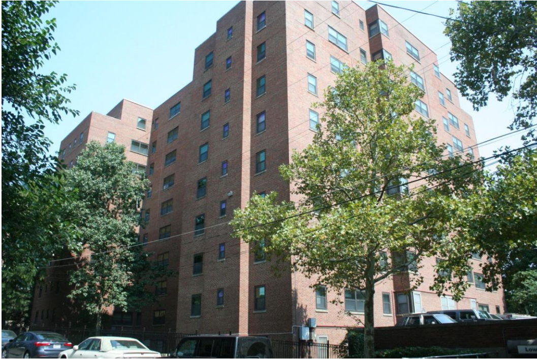
3700 Reading Road, South and Rear (East) elevations
