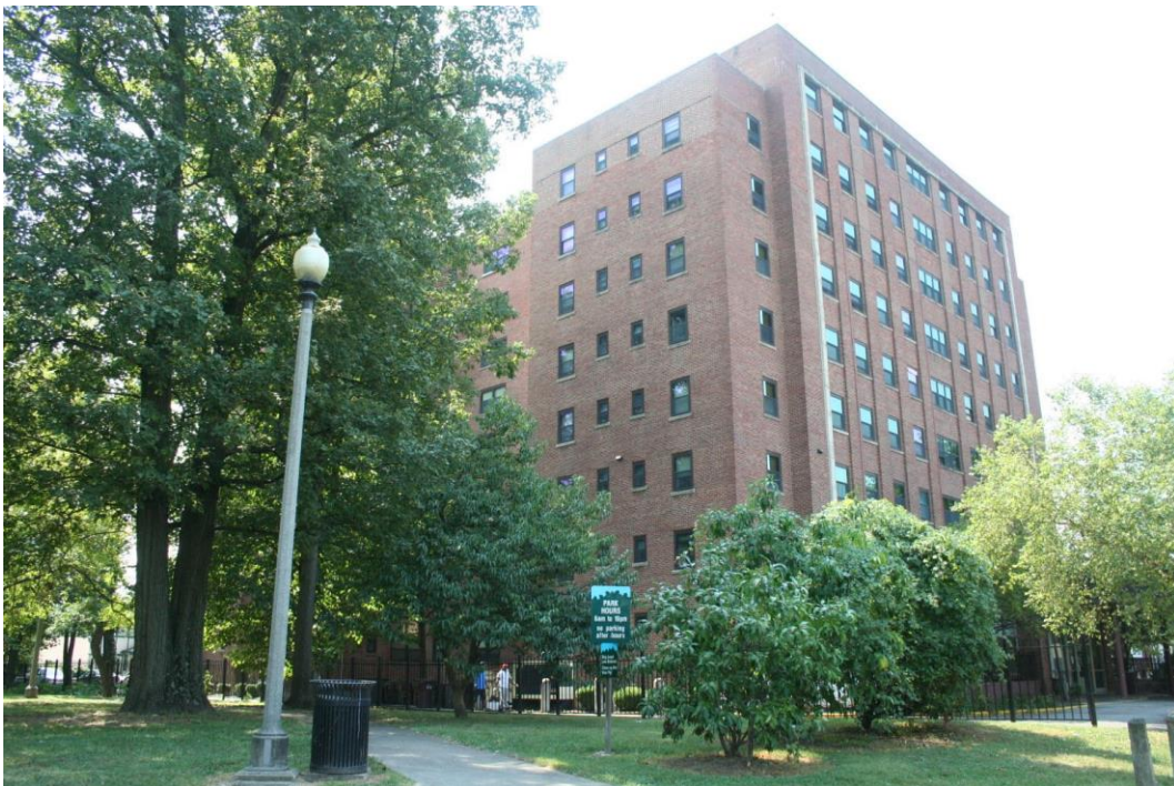
3700 Reading Road, North and East (Front) elevations
