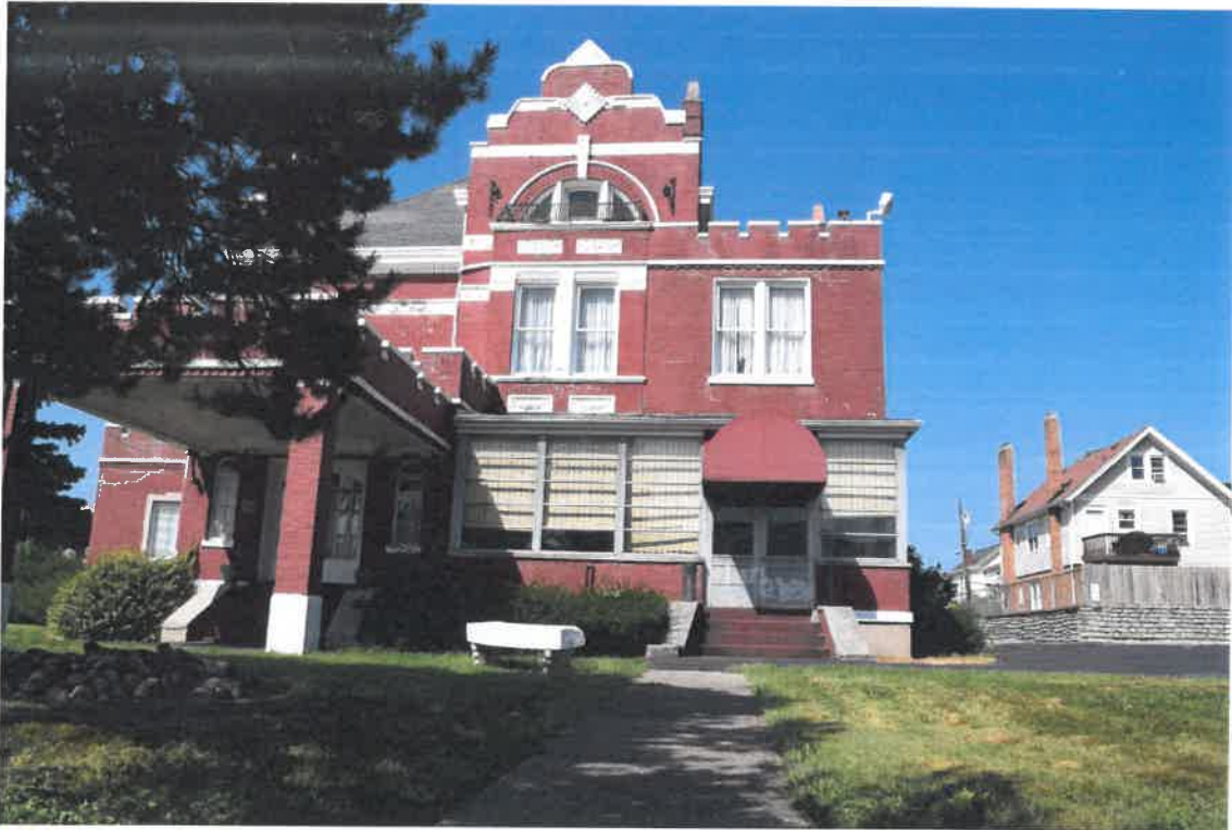
Figure 9: View of east elevation, August 23, 2021.
