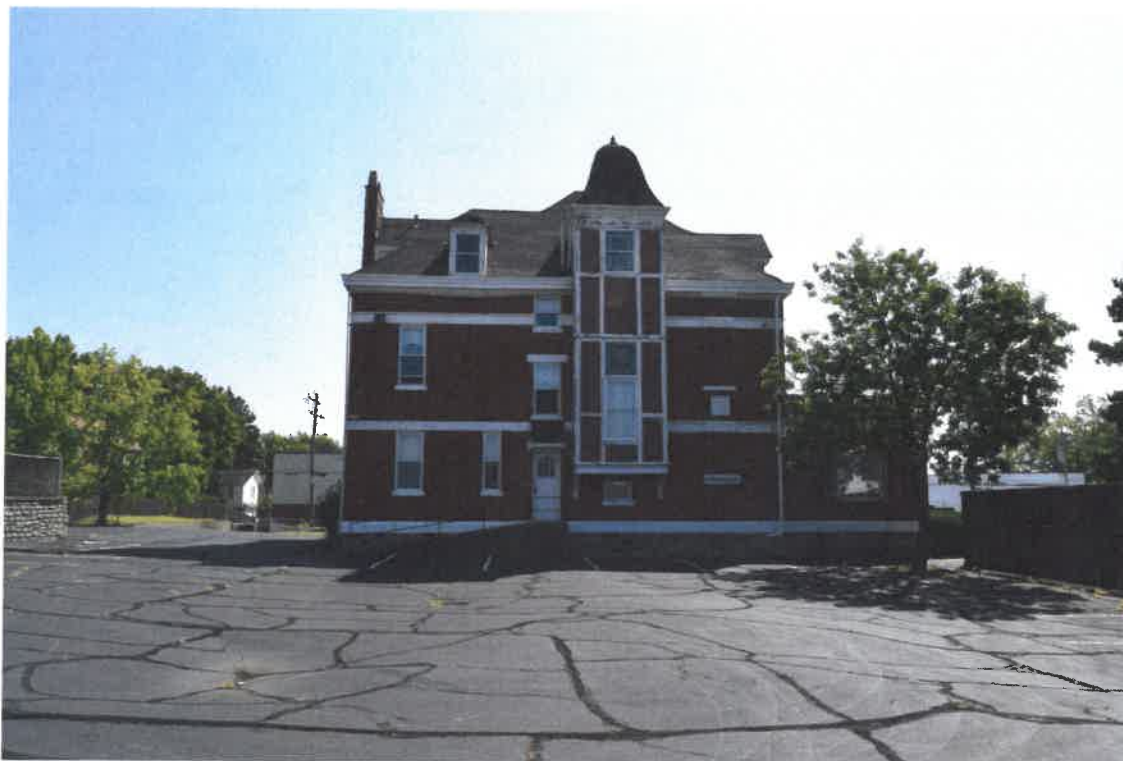
Photo 10: View of west elevation, August 28, 2021.
