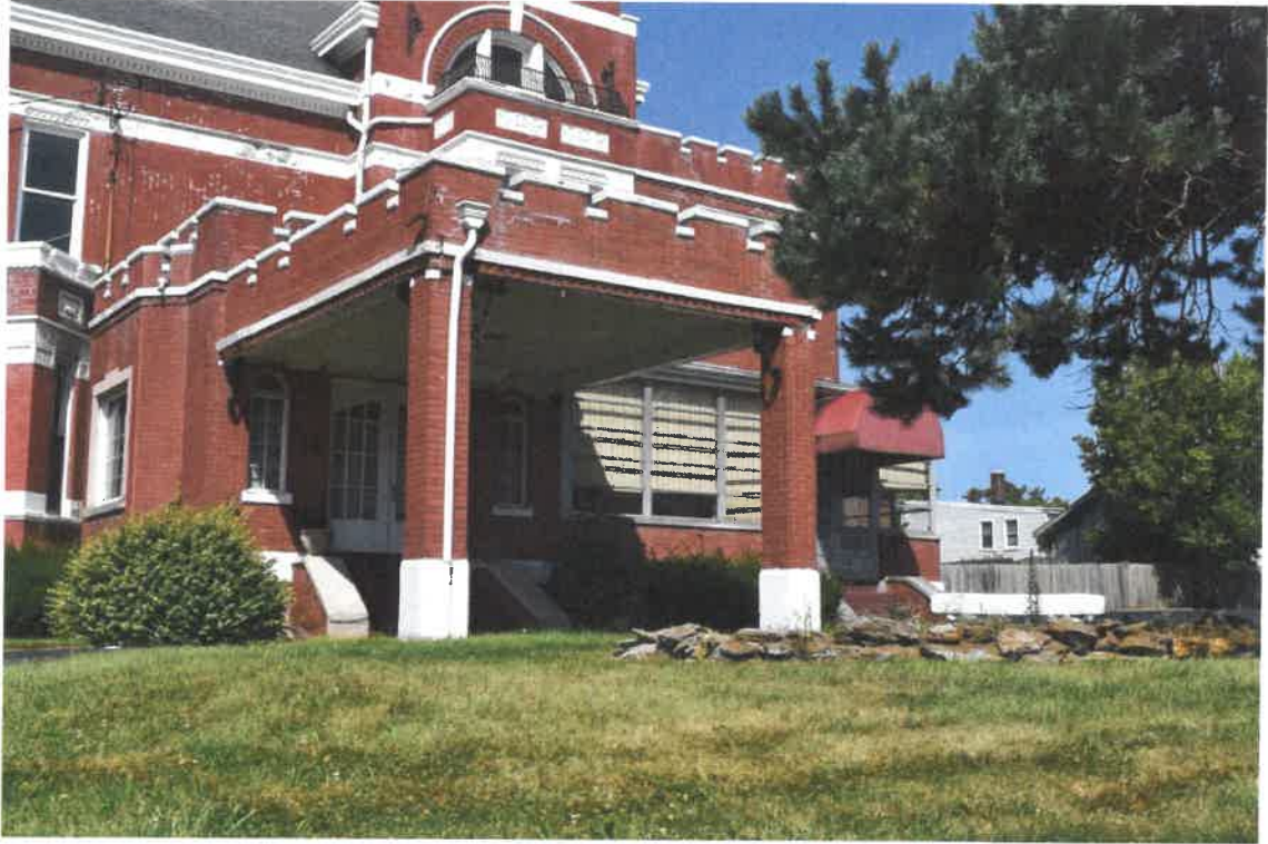
Photo 14: Detail of porte-cochere, August 28, 2021.
