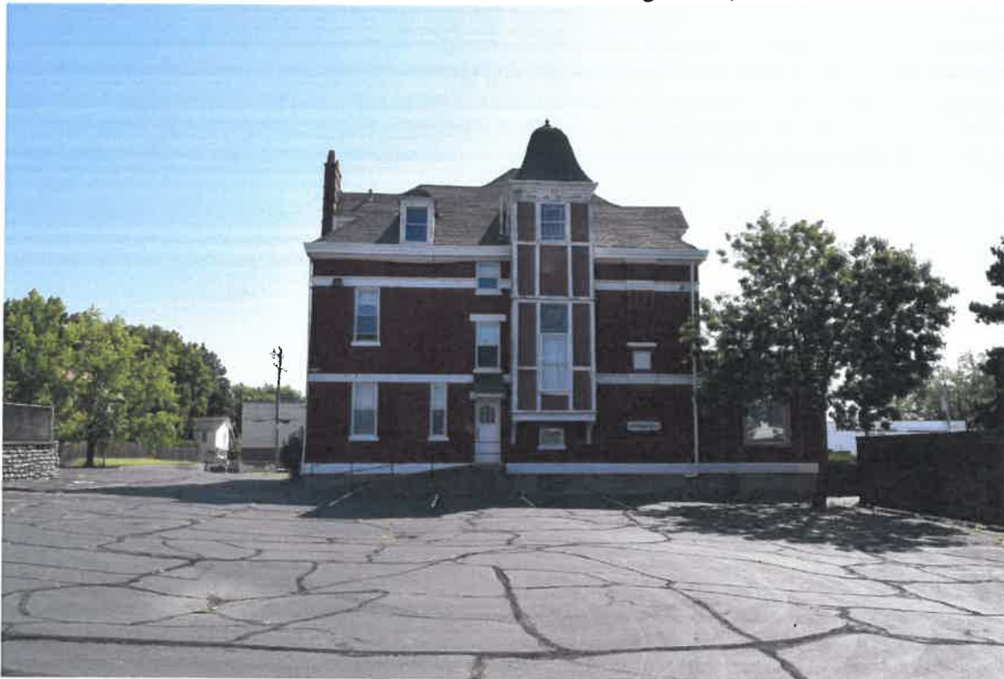
Photo 10: View of west elevation, August 28, 2021.
