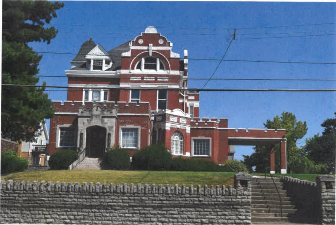
Figure 8: View of primary (south) facade, August 23, 2021.
