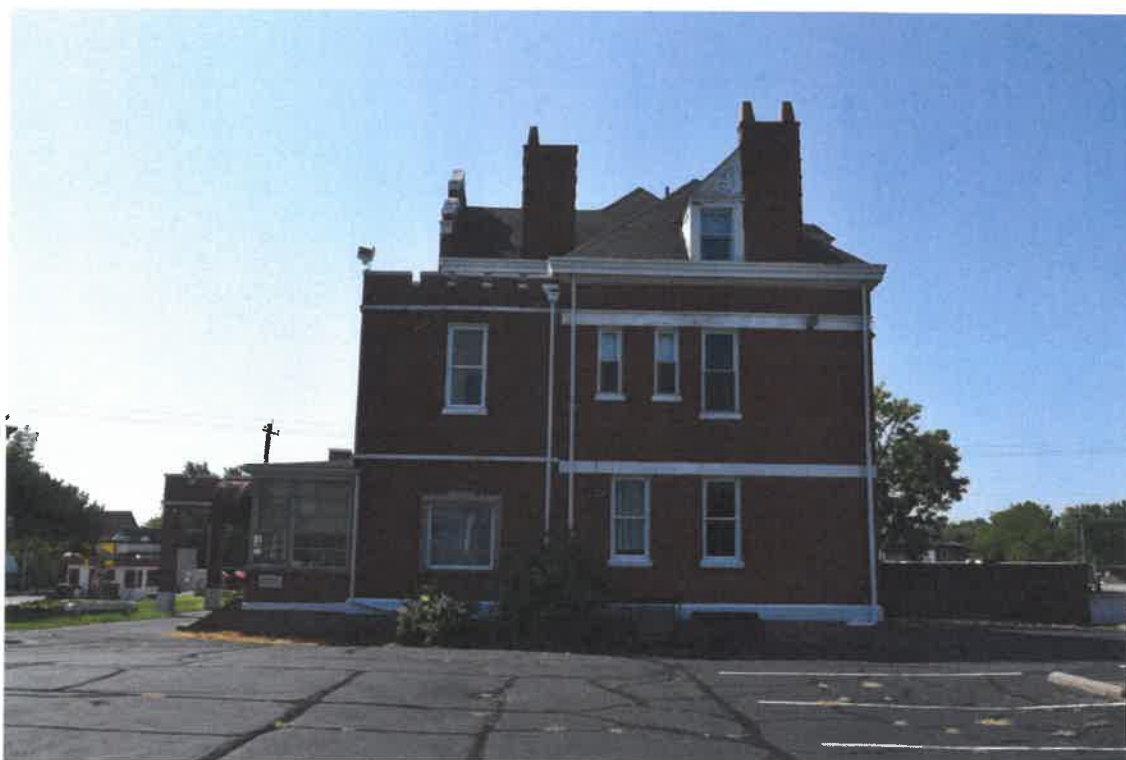
Photo 11: View of north elevation, August 28, 2021.
