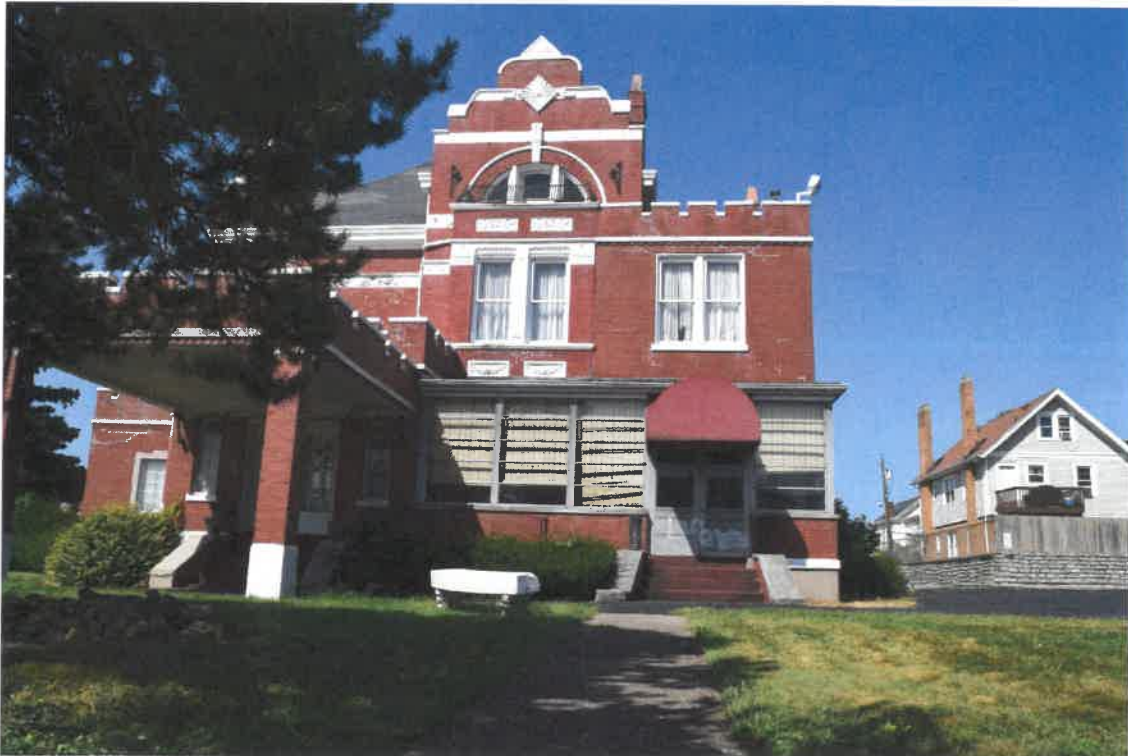
Figure 9: View of east elevation, August 23, 2021.
