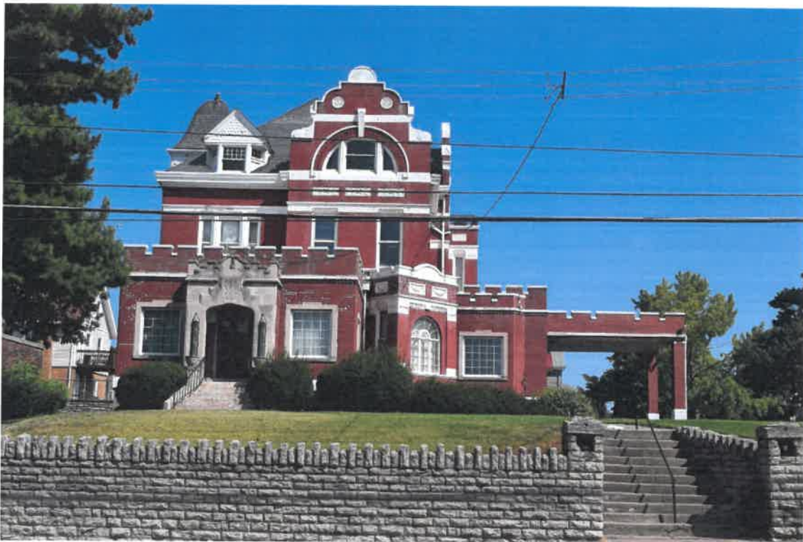
Figure 8: View of primary (south) facade, August 23, 2021.
