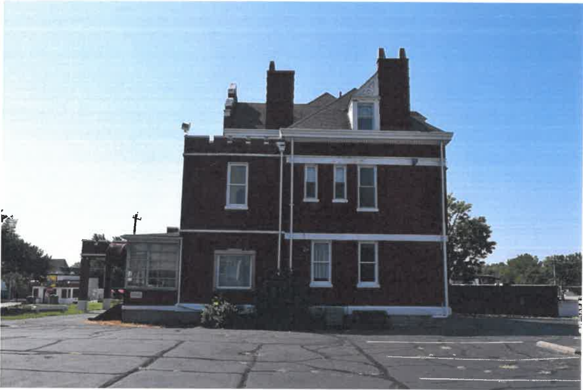
Photo 11: View of north elevation, August 28, 2021.
