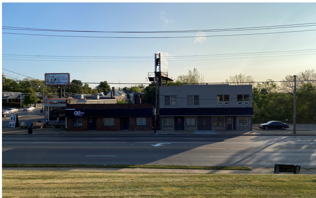
Redevelopment opportunity at the corner of W. North Bend and Colerain Avenue (5400 Block)
