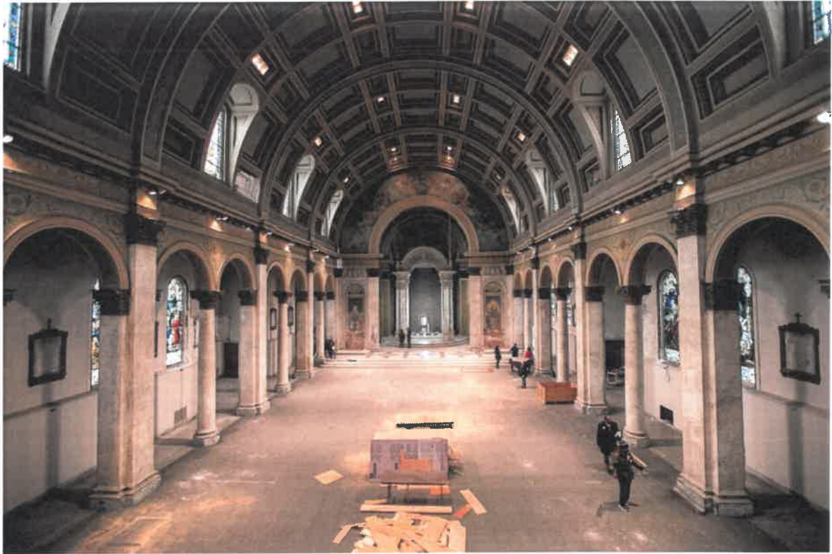
Figure 7 View of interior of church from choir loft, depicting arcaded side aisles and barrel-vaulted, coffered ceiling.
