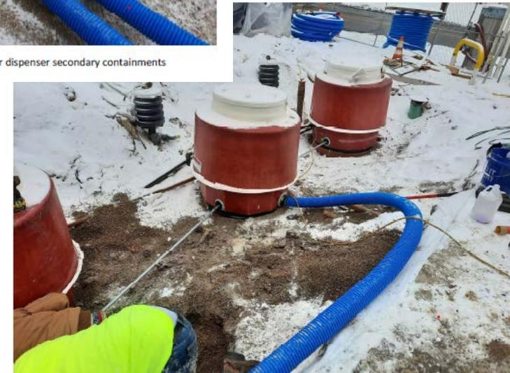
Installation of Fuel Pump Secondary Containments and Spill Buckets
