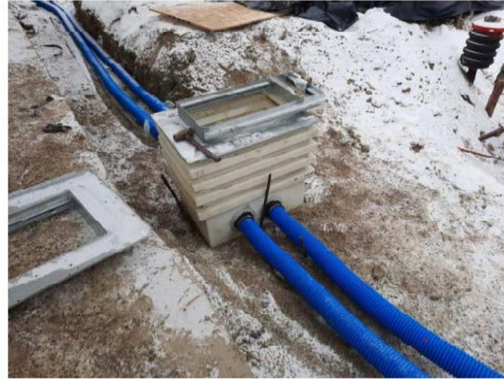
Installation of double wall product piping and under dispenser secondary containments
