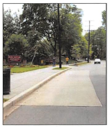
Figure 31: Example of Concrete Bus Pad
