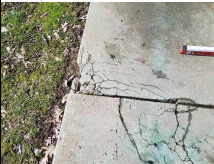
11. French Park cracked sidewalks
