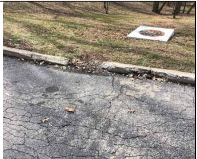
8. Eden Park damaged curb
