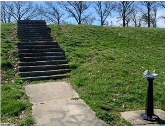
15. Mayfield steps with no handrails
