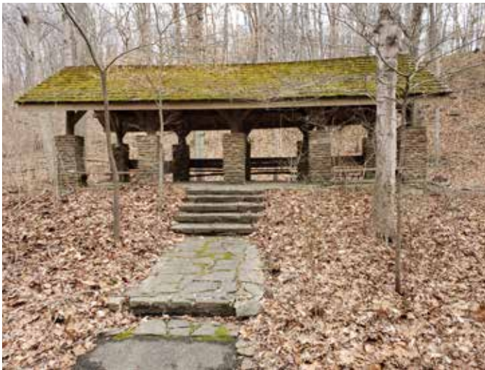
13. California Woods sagging roof on shelter
