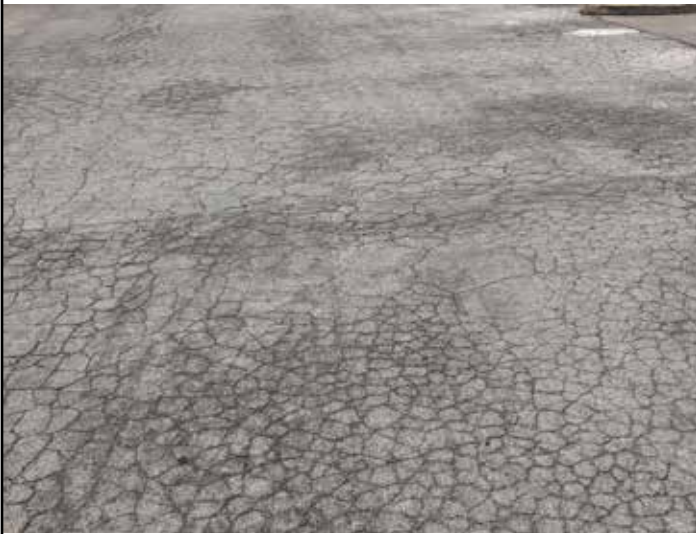
9. Sawyer Point deteriorated asphalt
