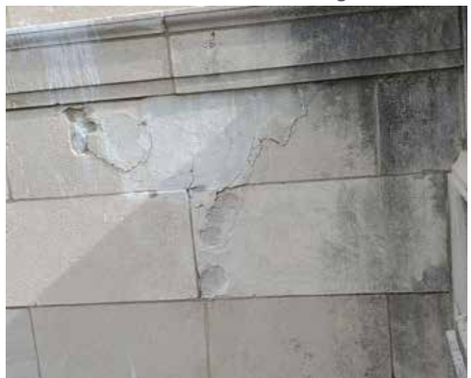
24. Ault Cascade delaminating sandstone
