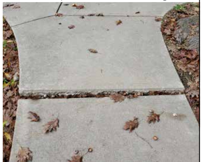
12. Kennedy Heights uneven sidewalk
