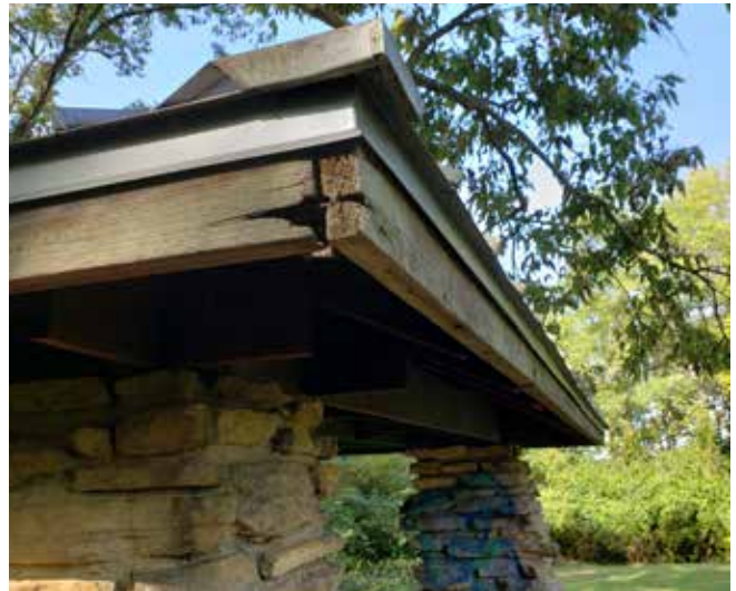
22. Mt. Echo shelter roof damage
