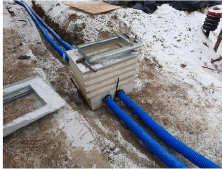
Installation of double wall product piping and under dispenser secondary containments
