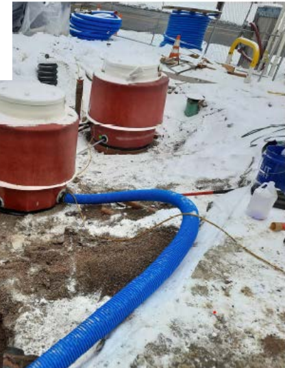
Installation of Fuel Pump Secondary Containments and Spill Buckets
